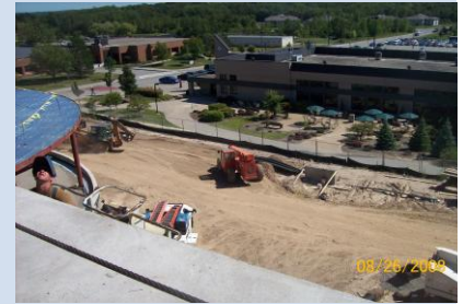
Silt fences around the project site controlling erosion
