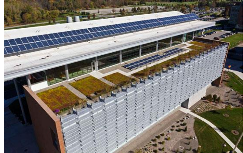
Figure 12: Solar array on roof of Sustainability Institute Hall
